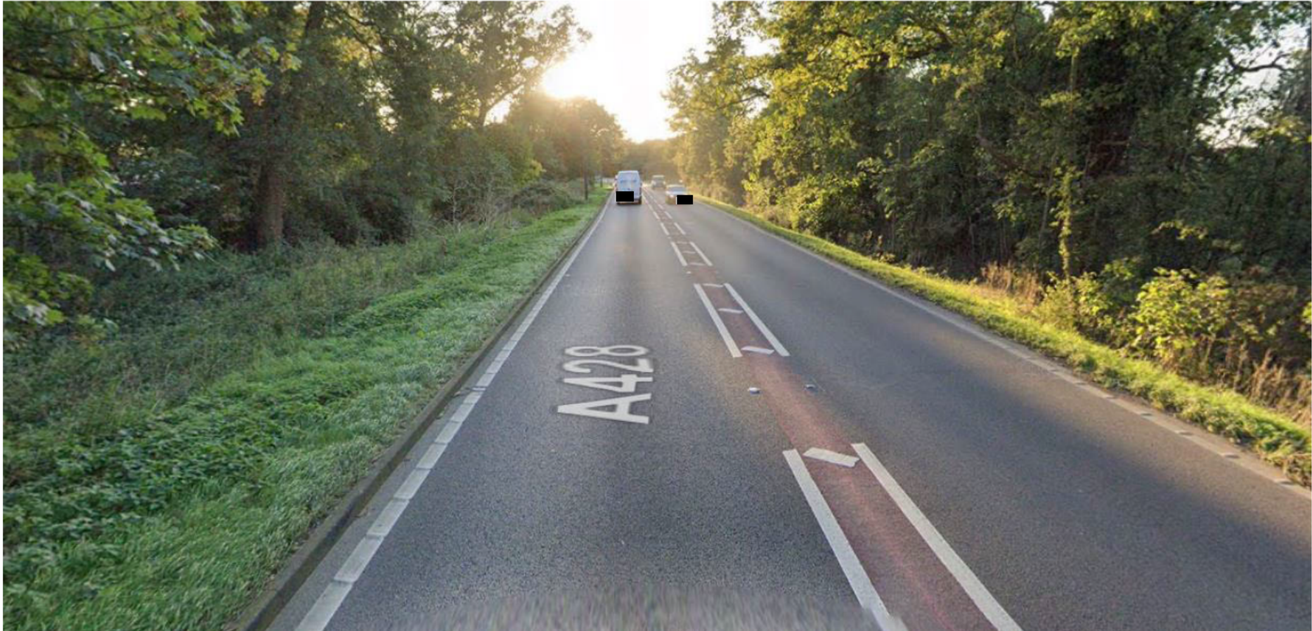
Figure 13: Existing A428 looking west. Wider verges
