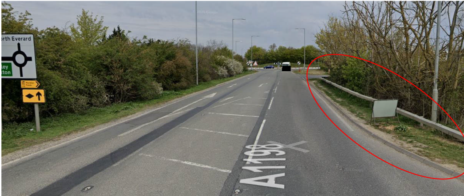
Figure 3: A1198 south of Caxton Gibbet junction with A428, looking north. Reference 1
